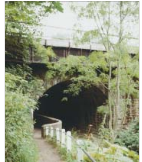
Below right: a view of the road bridge carrying the A359 over the railway. The abutments on the down side are the original stone ones. Those on the up side were built of engineers brick when the formation was widened to four-track.
