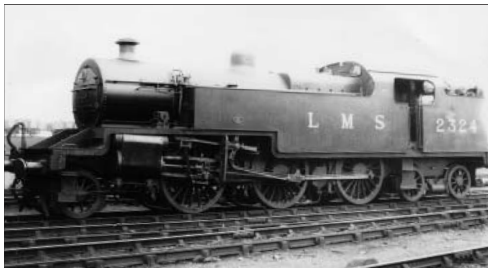
Above: captured in the 'first flush of youth' is Fowler 2-6-4T No.2324, at Derby shed on 22 July 1928. Note lack of outside steampipes, and brakes on the pony and bogie wheels. Last of the first batch of 25 machines (as represented by the drawings), the locomotive was exactly a month old when photographed. Photo: W.G.Boyden, courtesy Frank Hornby.
