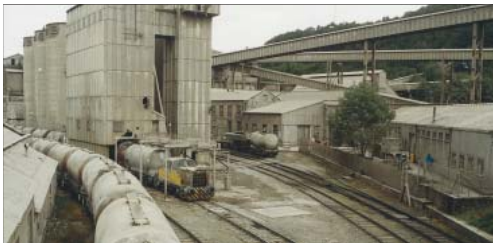
Left: Sentinel Derwent, a 1960s-era shunter rebuilt in the 1990s by Andrew Barclay, is framed by the loading complex in this view of the Blue Circle Cement Hope Works. Just look at the spans of those covered conveyors!
